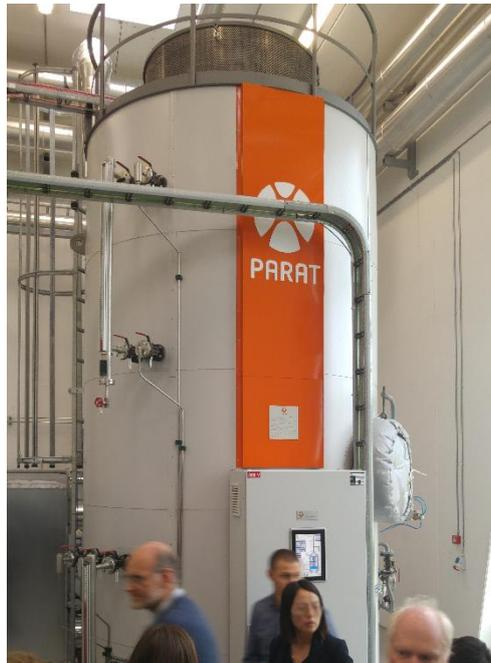
Figure 1: Electrode boiler (10 MW) at a district heating plant in Denmark (source: C. Doczekal)
